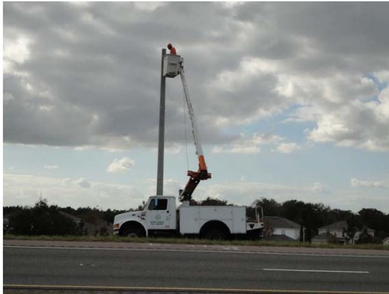
The Contractor for the Phase VIII Project, I-295 between I-95 and I-10, has continued with conduit installation and has installed several of the structures for the Dynamic Message Signs (DMS).
