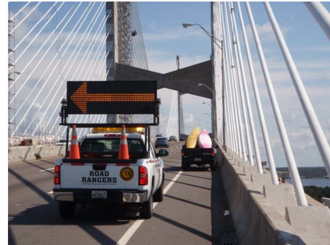
Road Rangers helping out on the Dames Point Bridge
